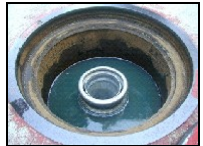
Spill bucket that contains liquid
