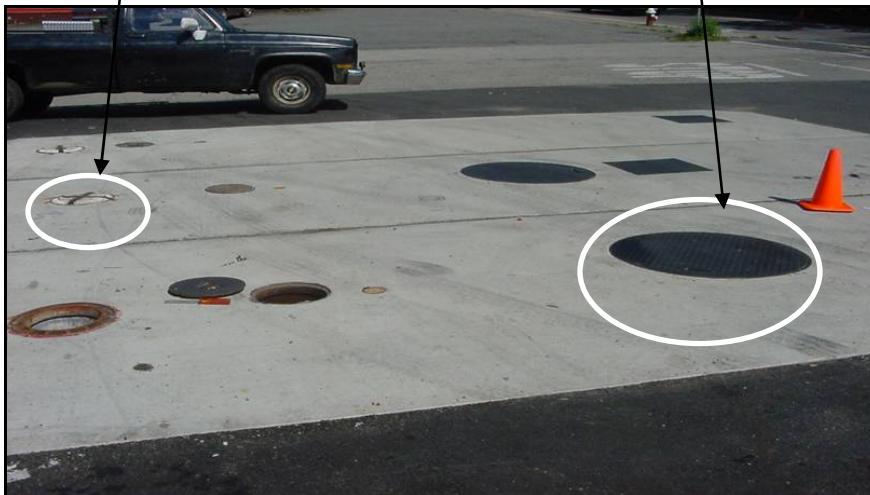
View of sump lids
