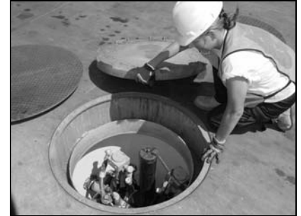
Person wearing safety gear while inspecting a sump
