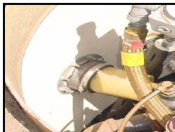
Sump penetration seals in good condition
