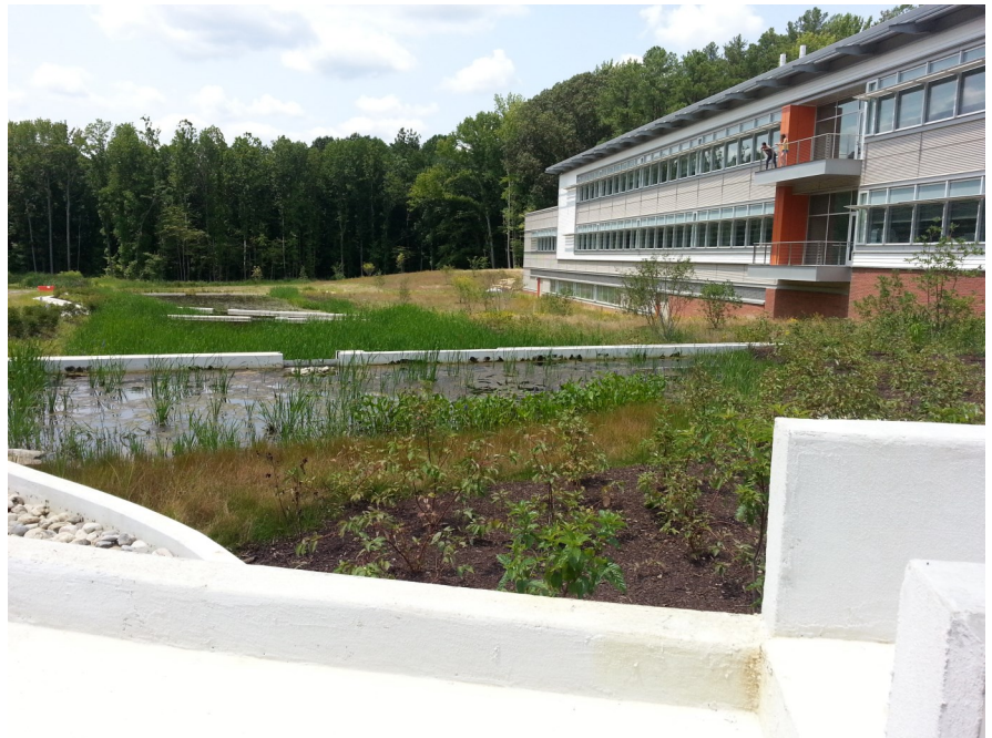
Teaching and Tranquility Rain Garden. This 4.56-acre constructed wetland filters stormwater and provides habitat for native wildlife. Rainwater from three cisterns and recycled gray water from the lab provide irrigation for the plants. Directly beneath it, a geothermal well field powers heating and cooling for the building. (Photo by Monaca Noble/SERC)
