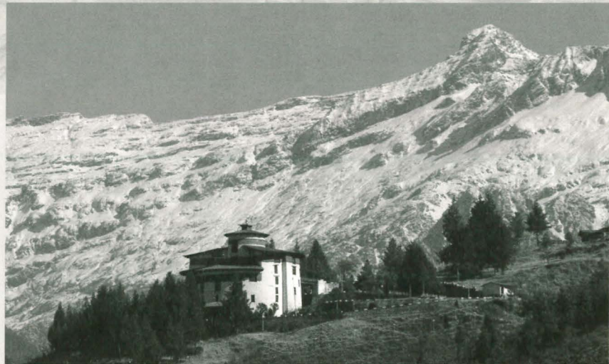
Bhutan's National Museum is housed in the historic Ta Dzong (watchtower), which is nestled in the hills above Paro Dzong. Its rounded, shell-shaped walls are an impressive accomplishment of seventeenth-century Bhutanese architects and builders. Photo copyright Michael Tobias
