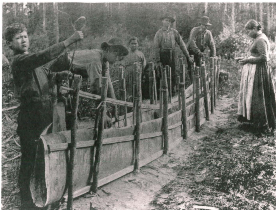
Canoe building required several people working together. Here the bottom bark is held down by a frame weighted with large stones in preparation for sewing the bark with split spruce roots. The seams are then sealed with pine or spruce pitch mixed with deer tallow. Photo courtesy Michigan State Archives, Department of State
