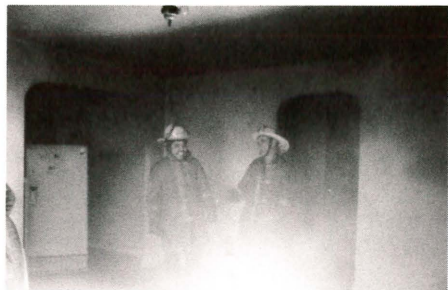
7 Talking it over on the fire ground
