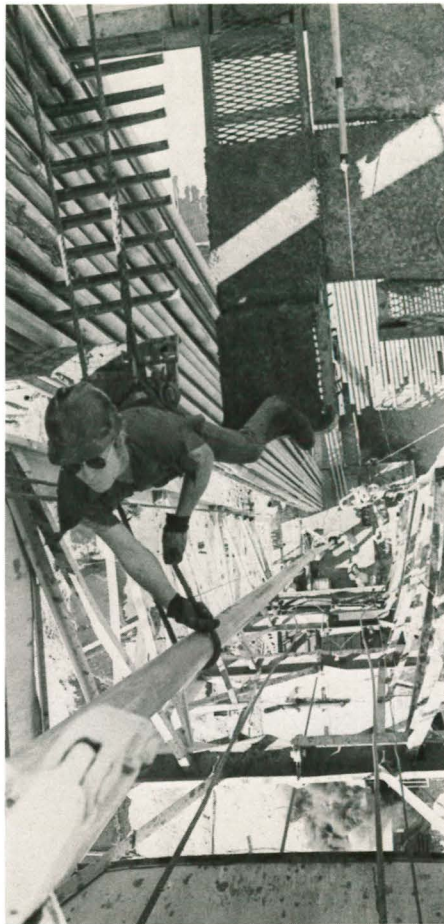
A derrick or "monkey" man works high above the drilling platform. Photo by David Moody © 1978.
